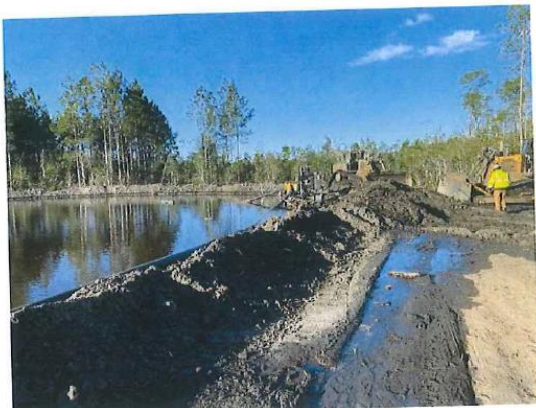
Northwest corner Reclamation cell (January 31, 2024)
