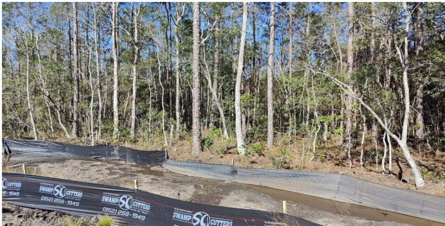
Area 1, showing double row of silt fence containing standing water.
