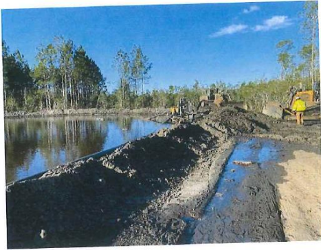
Northwest corner Reclamation cell (January 31, 2024)
