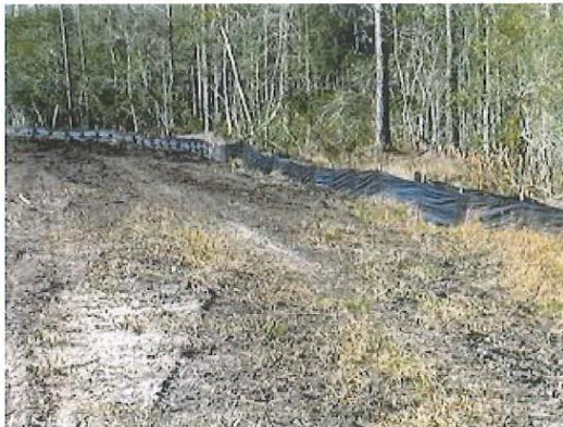
Silt Fence Repaired (January 31, 2024)
