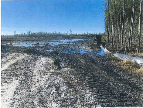
Area 2 Water on Topsoil return area (January 31, 2024)
