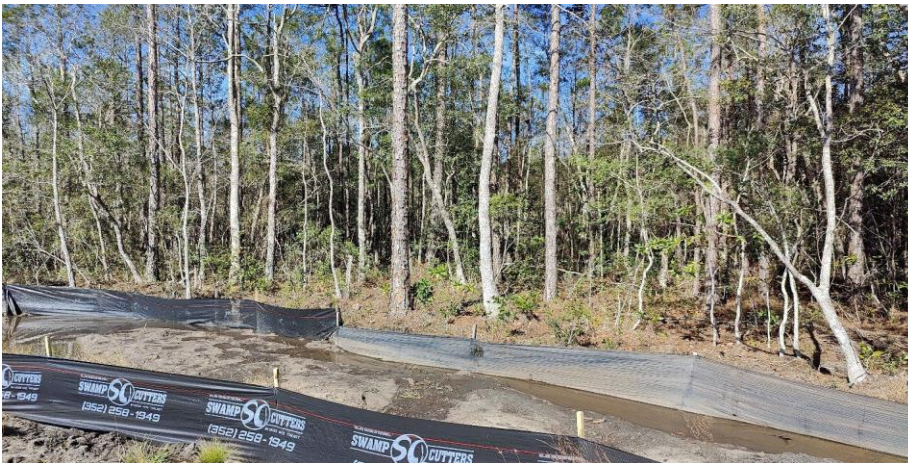
Area 1, showing double row of silt fence containing standing water.
