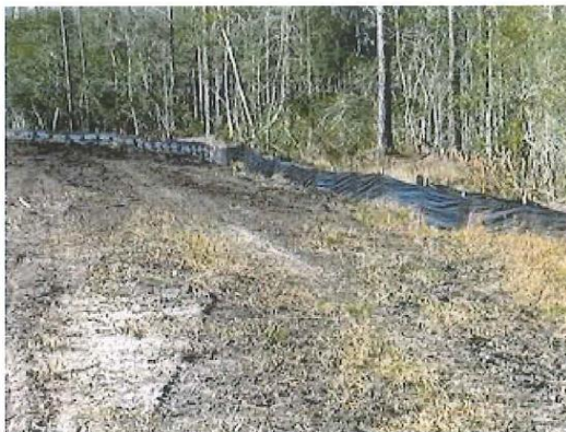
Silt Fence Repaired (January 31, 2024)
