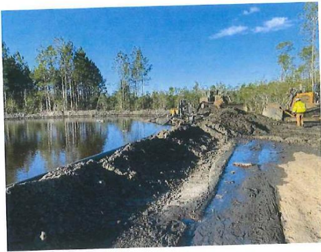
Northwest corner Reclamation cell (January 31, 2024)
